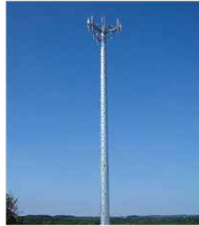
(3) Tower 1 kaki / Pole
